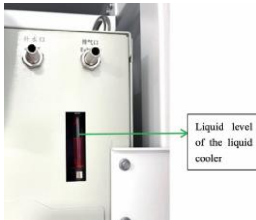
Figure 6.3 Liquid Level of the Liquid Cooler
